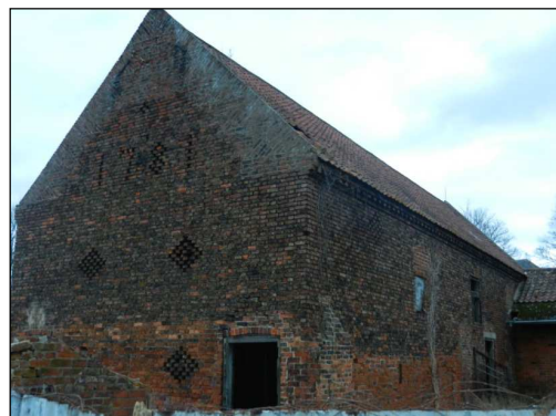
Fig. 33 Barn of 1781 on the site of Horkstow Manor. Diaper pattern ventilation holes in the gable-end wall, dentilled pattern brick ornamental course below eaves (no evidence of a threshing floor entrance).
