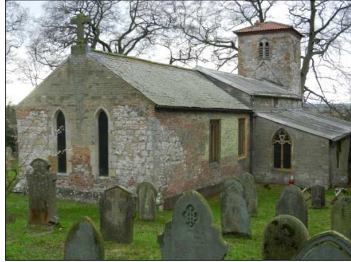
Fig. 21 Horkstow church as seen from the north-east section of the churchyard. In the east wall of the chancel two restoration lancets have been set into a chalk and early brick wall, the bricks probably being used to replace decayed chalk blocks. Above, a coursed limestone restoration wall dating from when the chancel roof was raised. The medieval roof-line of the nave is shown in the east walling of the tower and the limestone ashlar of the north aisle and its stylised window tracery date from the 1895 restoration.
