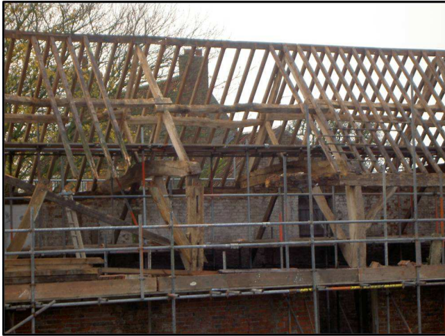
Fig. 38 Photograph taken c. 2012 and showing the late-medieval/early-modern(?) barn just north of Horkstow Hall which has undergone an extensive and long running programme of restoration. The large timbers of the skeleton shown comprise adze-shaped tie beams, wall-posts and braces (angled) while the roof timbers comprise rafters linked to the ridge-board and supported by purlin boards.
