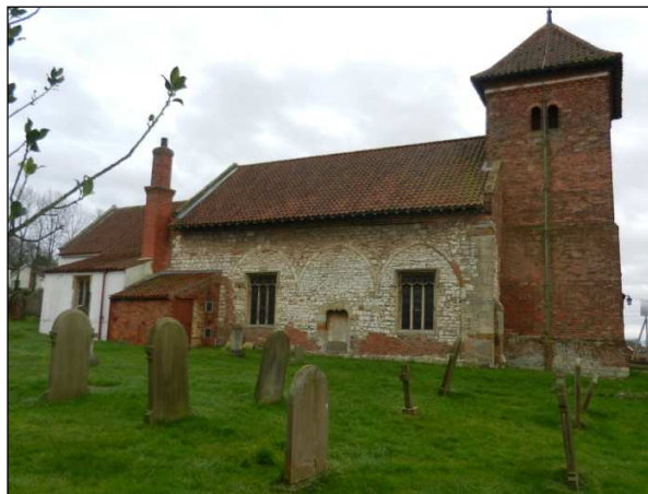
Fig. 22 Bonby church, viewed from the north. When an early north aisle was demolished coursed chalk walling was used to infill the arcade. These chalk courses are not continuous with those of the wall above and in the spandrels as this walling dates from the construction of the aisle. The arcades were originally built in a transitional style of the late 13 th century.
