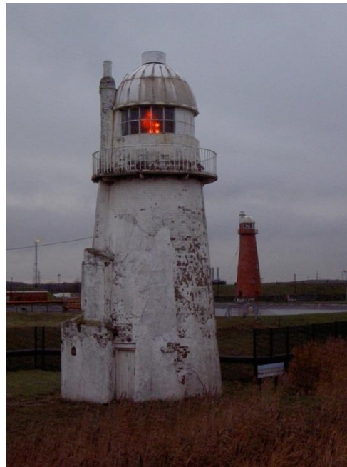
Fig. 23 The two 'leading lights' of Killingholme Marsh, built in 1835. The lower light seen in the foreground (still having a light) showing evidence of the staircases by which the 'keeper' and his family accessed their home. Two hundred yards away the 'upper light' was more like a traditional lighthouse. Both were built of brick, one painted the other rendered. By lining-up the two lights mariners sailing up the Humber could navigate the deep-water channel.
